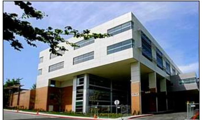
Providence Regional Cancer Center opens Monday in a new $62.4 million building in Everett that will offer patients a variety of treatment options.
